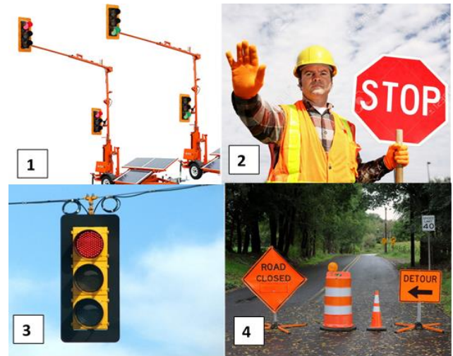
Figure 5: Alternative Competitors (1) Mounted Temporary Traffic Light, (2) Personnel on Road, (3) Flashing Red Light, (4) Closing Road
